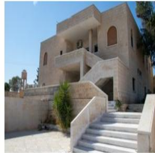
End of Restoration Work at St. George Monastery in Muhardeh
