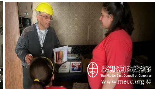
Assessing the apartments in each building to examine any cracks or damage
