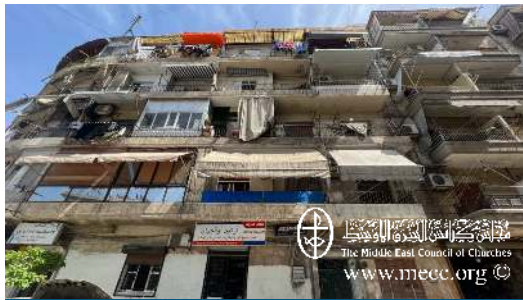
One of the building under assessment by MECC technical team
