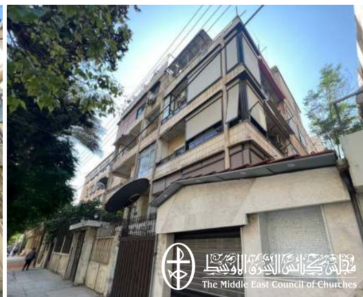
First building that will retrofitted
